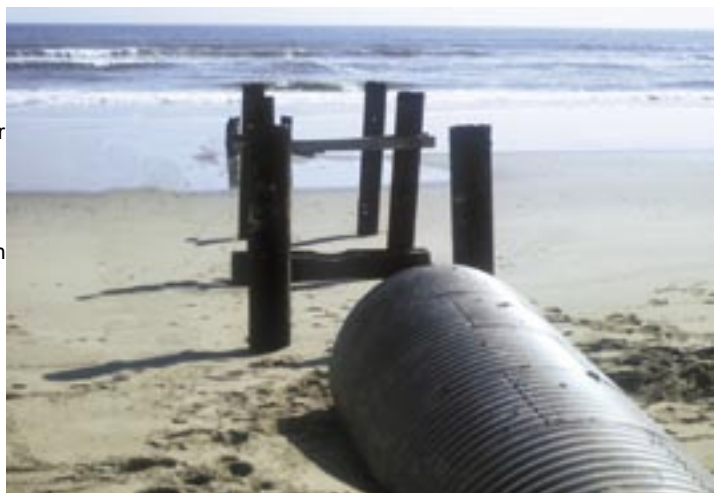
Aluminum pipe can be installed in salt water environments. (See Superior corrosion resistance section above.)
