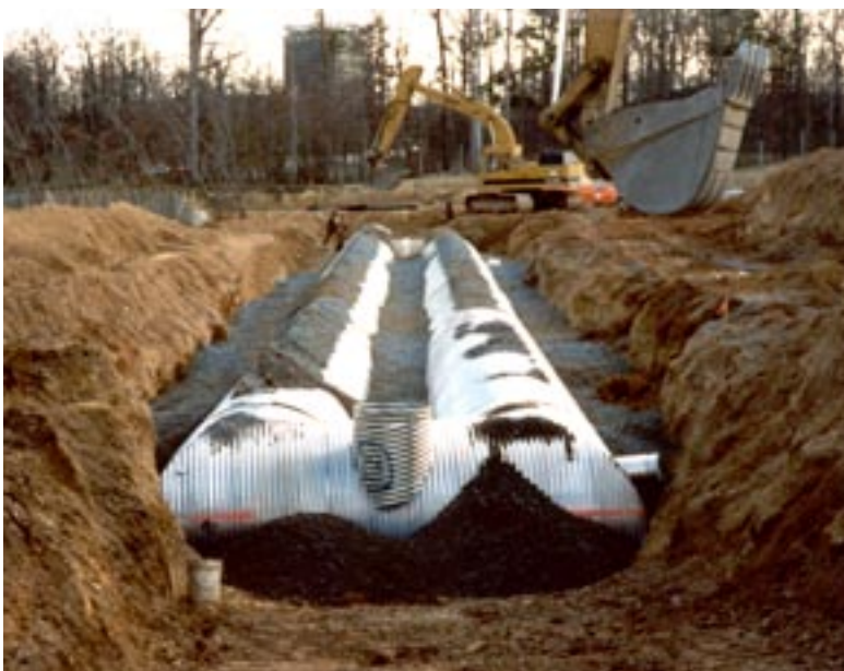
CORLIX Pipe cuts installation time and adapts well to a designer's detention/recharge system.
