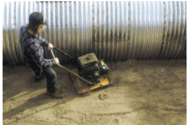
With proper backfilling and cover, CORLIX is an excellent choice for drainage pipe.
