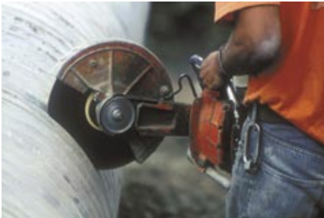
Aluminum Pipe is easily cut in the field.
