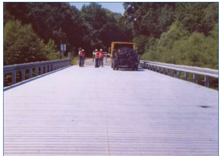
A continuous bridge deck
