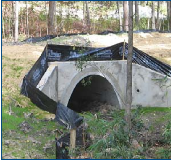
Preserves Natural Bottom - Lightweight modular arch units allow for a natural stream bed beneath roadways with minimal earth cover.
