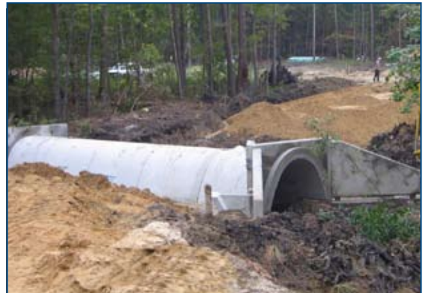
Precast Concrete Solution - Structurally efficient concrete arch provides the most waterway area per ton of concrete in the industry.
