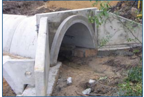
Strength of Arch - Unique shape capable of supporting heavy loads and high fill.
