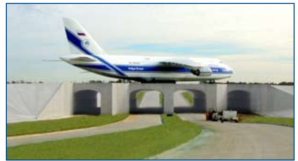
Taxiway bridge – runway expansion at Houston Intercontinental Airport supports 1.6 million pound payload
