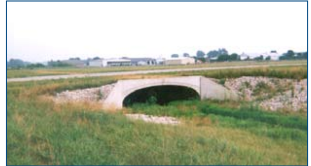
Stream crossing – allows continuation of runway over a stream cutting through the Greenwood Airport in Indiana
