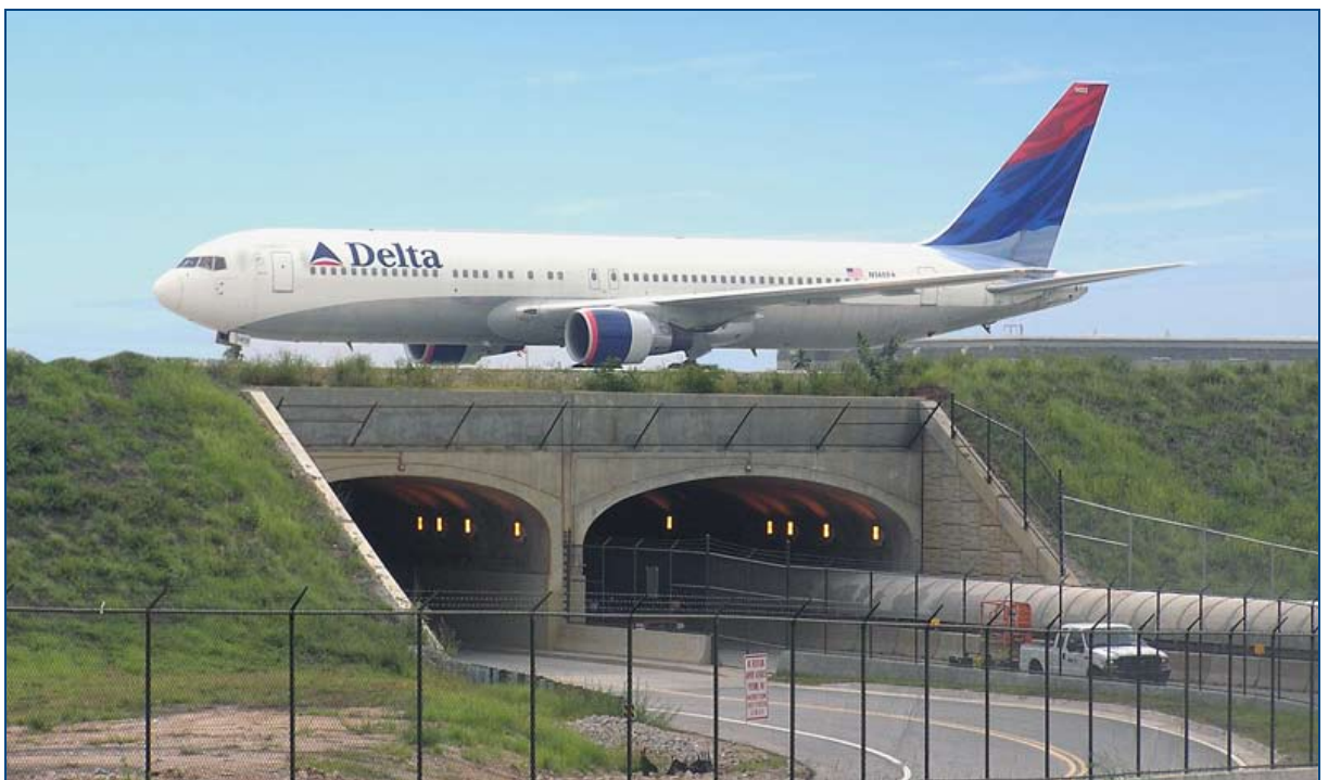
Runway extension – design supports aircraft loading on extended taxiway at the Hartsfield Atlanta Airport
