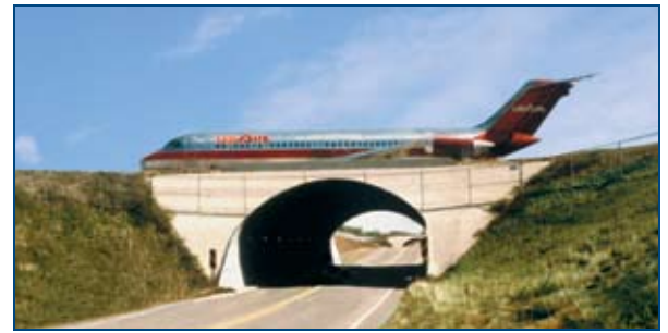
Taxiway overpass – SUPER-SPAN™ supports special aircraft design loading at the Port Columbus Airport
